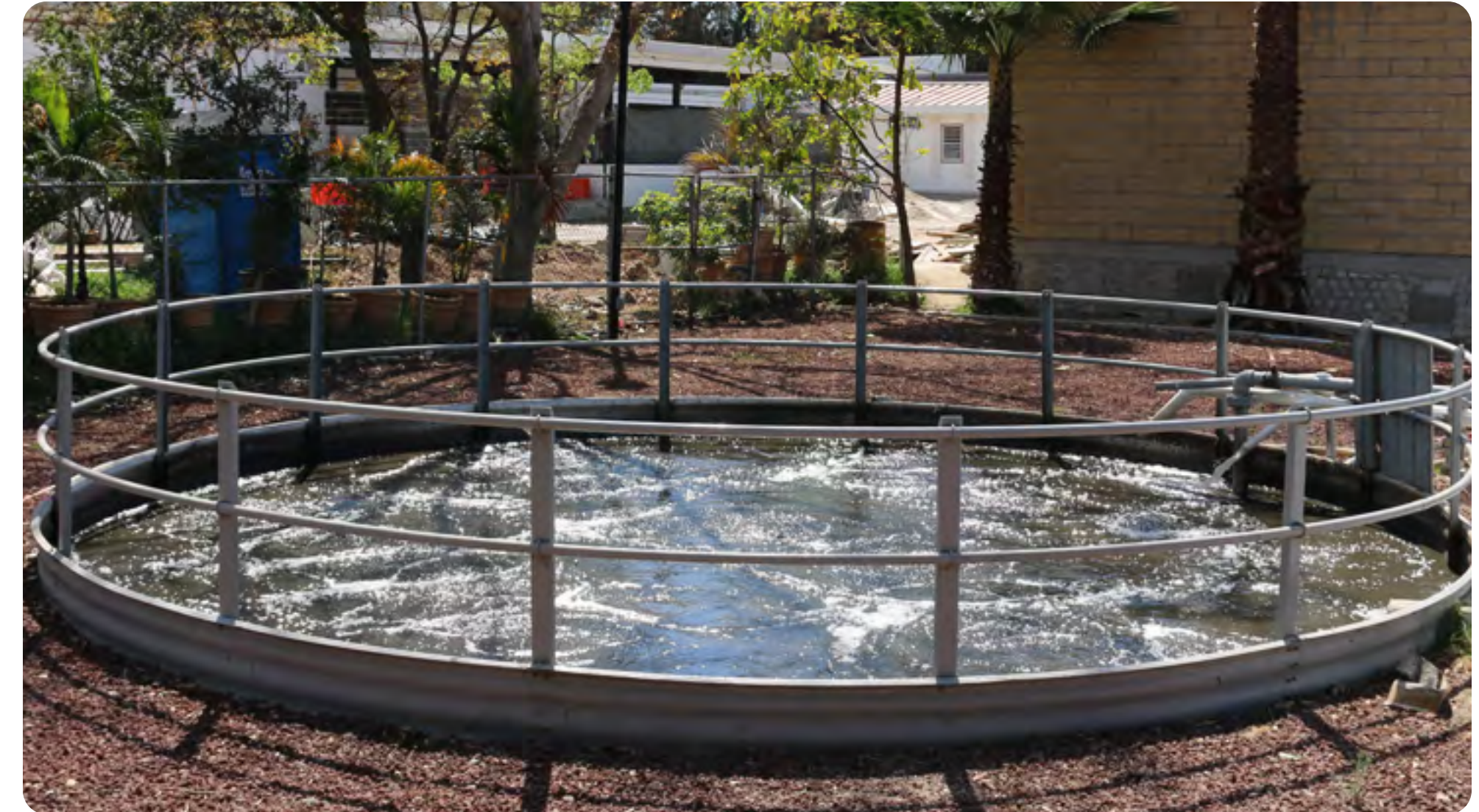
Wastewater treatment plant, Guadalajara Campus
