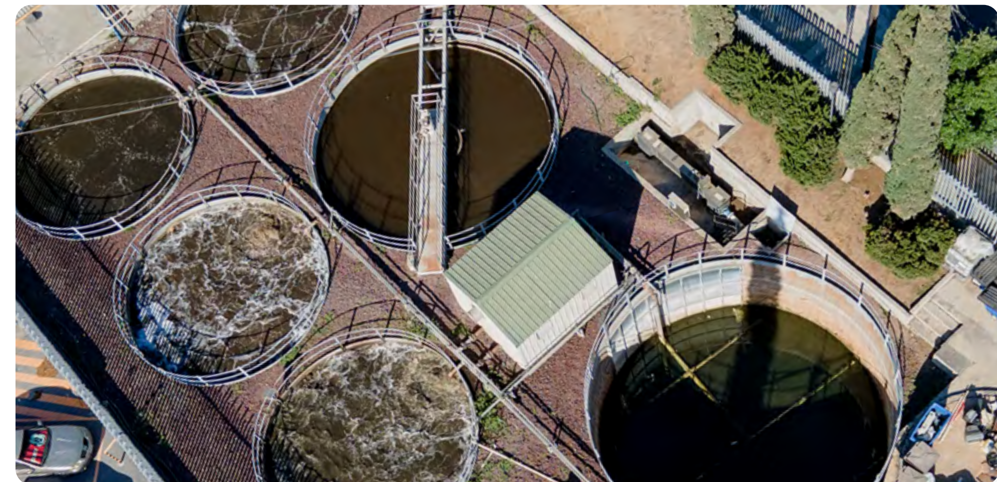
Wastewater treatment plant, Monterrey Campus
