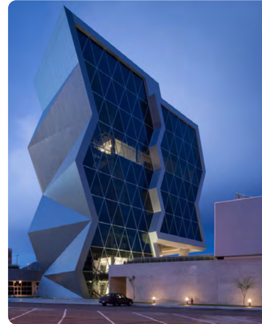
LEED gold certification of library, Monterrey Campus, and PITT (Innovation and Technology Transfer Park), Chihuahua Campus
