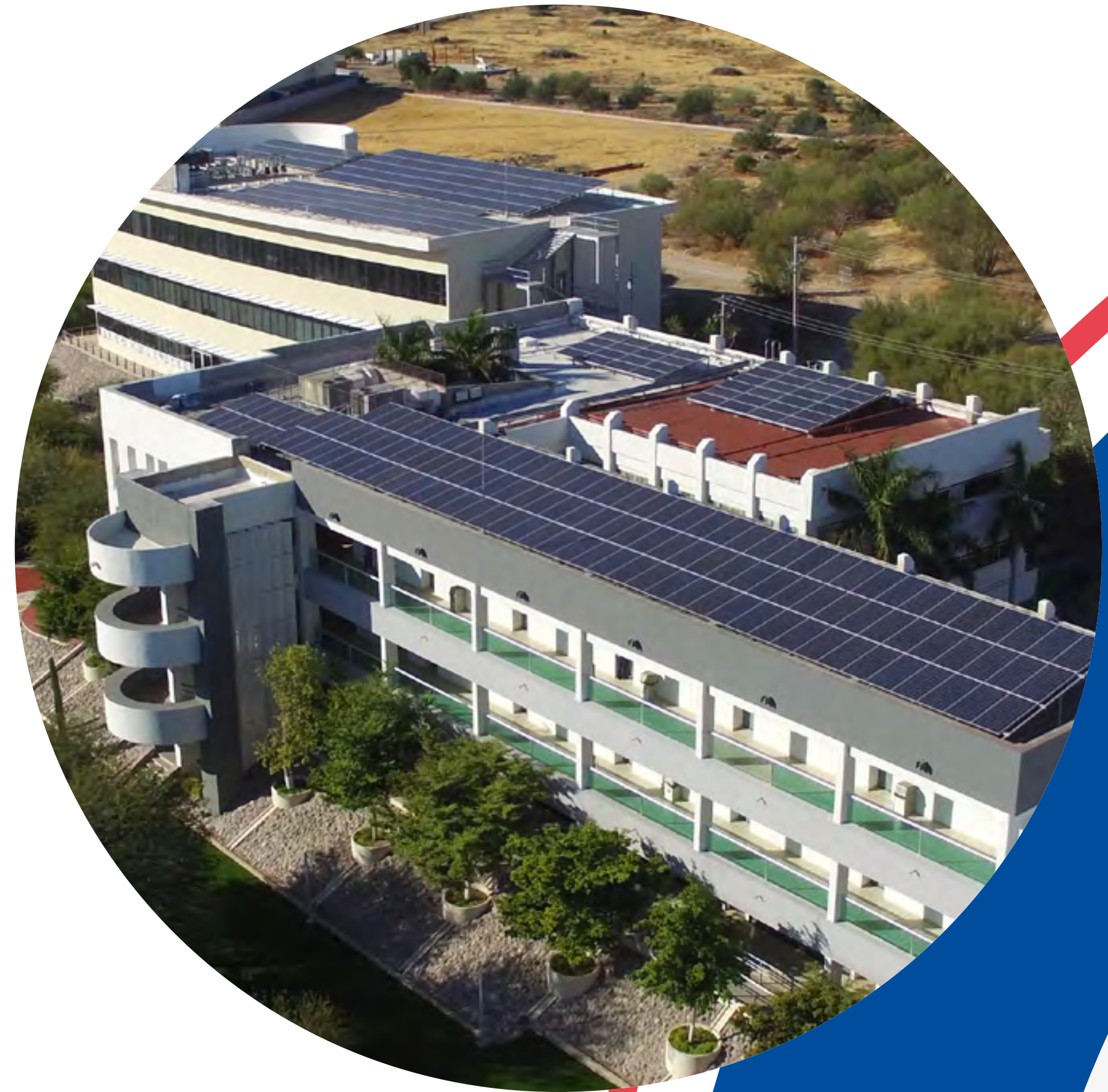
Photovoltaic Plant, Sonora Norte Campus
