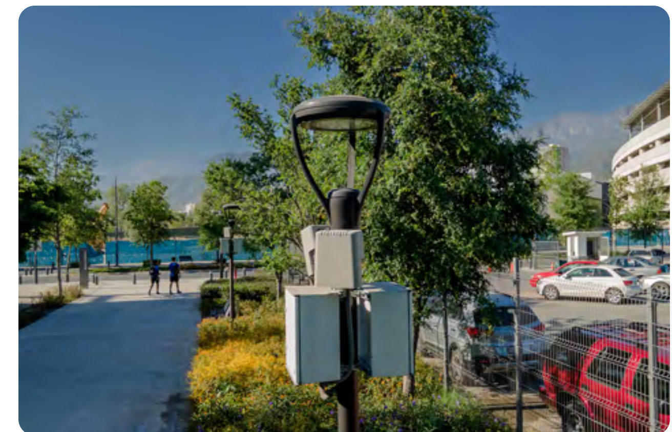
Photocells on lamp posts, Central Park, Monterrey Campus
